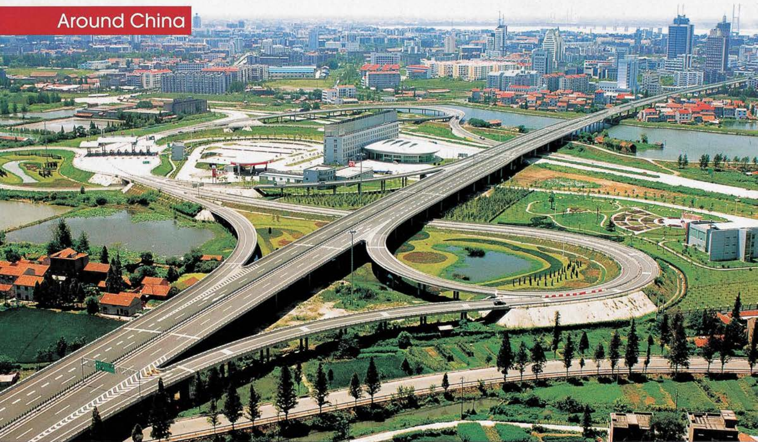
The Hubei section of the Erenhot-Guangzhou Expressway.
